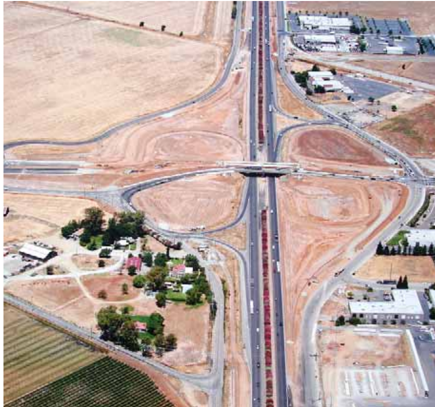
Aerial View of Grant Line Road – SR 99 Project.
