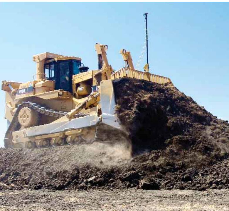
GPS Controlled D10 cuts turbines pads.
