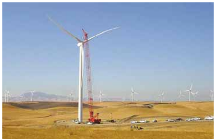
Mortensen's crane placed the wind turbines.
