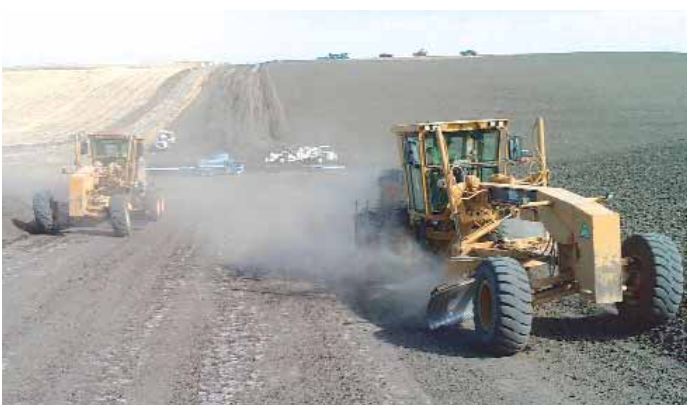
Grading the road to the turbines.
