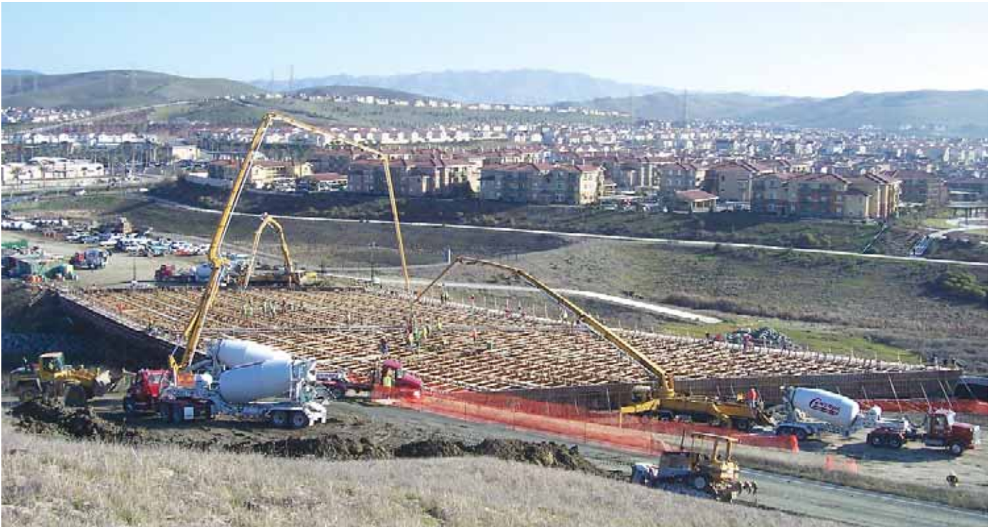
North bridge – 2,100 cy bottom deck and stem pour.
