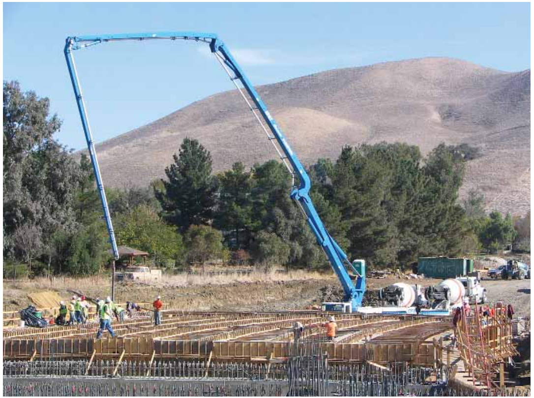
South bridge – 1,800 cy bottom deck and stem pour.
