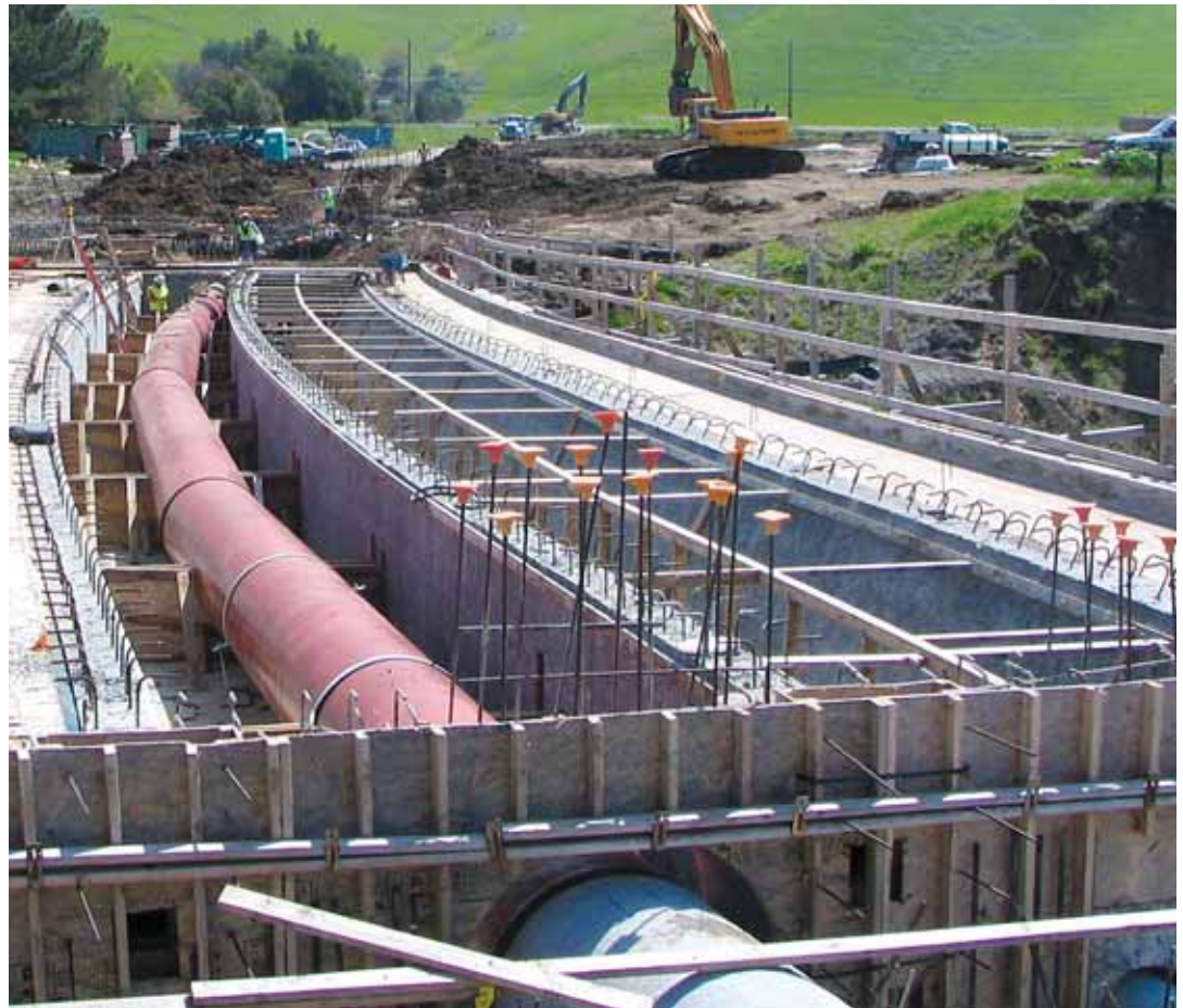
Welded steel pipeline installed by RGW underground crews.
